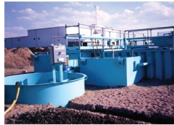
ADDIGEST Pet Food Production Plant - Mexico
